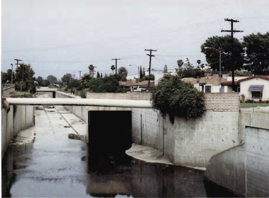
Picture 1: Ballona Creek during dry weather. This picture shows Ballona Creek at the Fairfax Street Crossing. The small flow visible at the bottom is dry weather flow.
