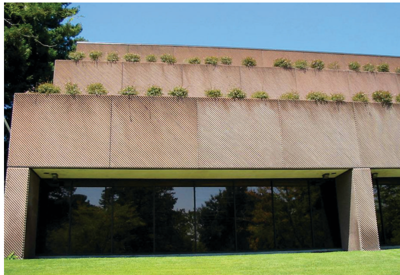
A government building in Santa Rosa where researchers tested the feasibility of using thermal mass to shift demand.
