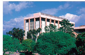
A library at UC Santa Barbara, one of five buildings statewide to test fully automated demand response.
